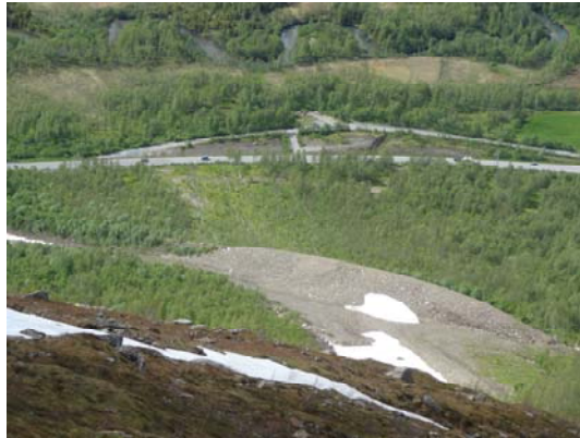
Photo 3: Hestvollan avalanche path with a leading dam. But still better protection needed for highway E8 crossing the run out zone. (Photo June 29 2012: O.A. Helgaas)
