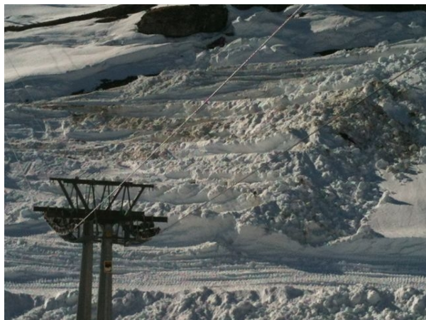
Fig. 6: Lungern-Schönbühl, canton Obwalden, Switzerland in January 2012: to reduce the danger from a full-depth avalanche, the slab was partially removed by snow removal machines.
