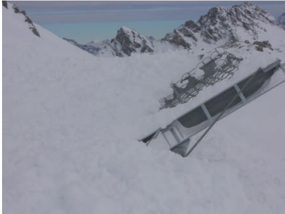
Figure 5. Filled up Snowcatcher after an avalanche event.
