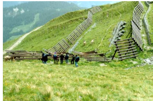
Fig. 3: Snow supporting structures destroyed by an avalanche, which was released high above the controlled area. The structural safety is not fulfilled for impacts of large avalanches. The reliability is low.
