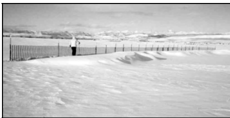
Figure 1. Interception and retention of snow in dense drifts is affected by snow fence design.
