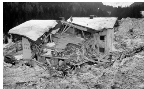
Figure 1: Photo of a house damaged by a snow avalanche in Valzur near Galtür, Austria, 1999, S. Margreth photo.
