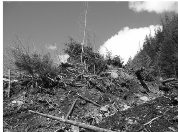
Figure 6: The run-up of the avalanche flow at Tower 39 was < 1m from overtopping the splitter.
