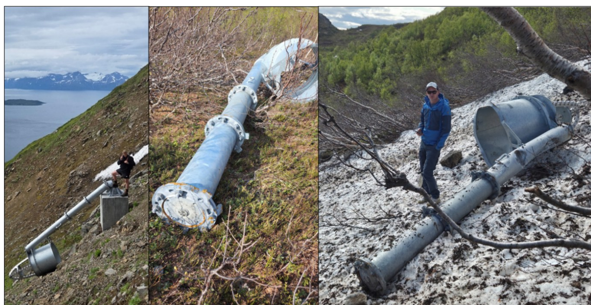
Figure 1: Damaged installations during the season of 2024/25.
