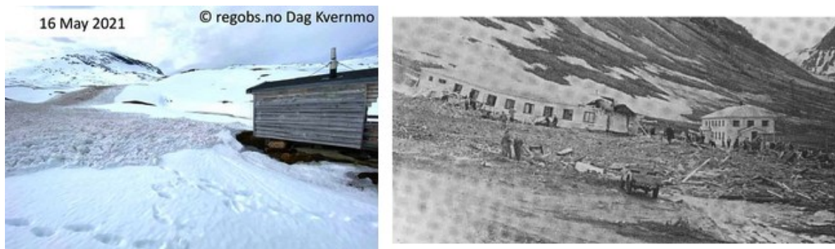
Figure 4: Slushflows present a significant hazard in the Arctic.: Right: Buildings in Haugen, Svalbard, that were destroyed by a slushflow in 1953 (Picture from UNIS 2006). Left: Slushflow observed near a cabin, note the shallow terrain and the long run out of the slushflow (Sund et al. 2024).
