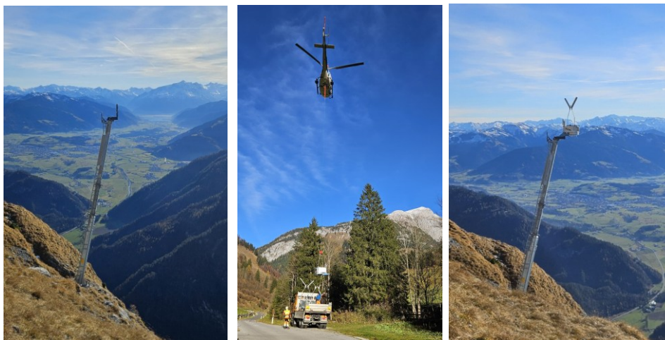
Figure 8: Wyssen avalanche towers without (left) and with the deployment box mounted (right); helicopter transport of a loaded deployment box (middle) to the Labeckbrunn avalanche towers in Saalfelden.
