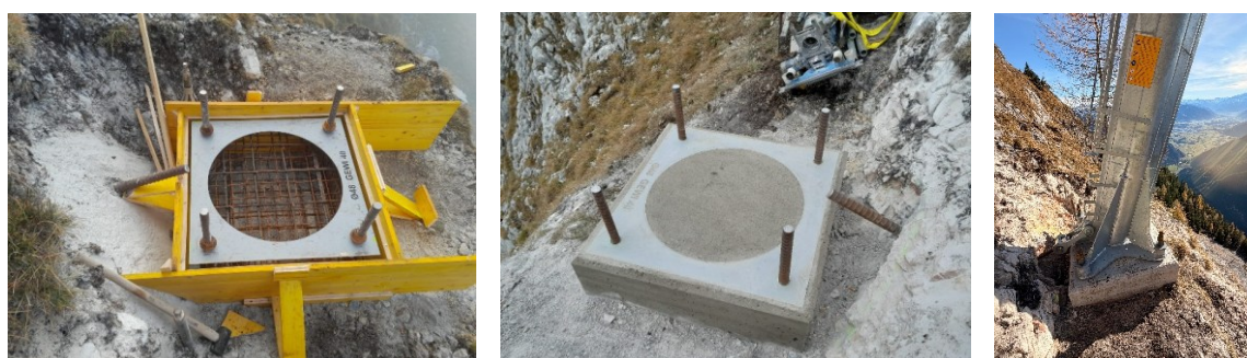
Figure 5: Tower foundation before pouring the concrete (left), after concreting (middle) and with the tower installed (right).
