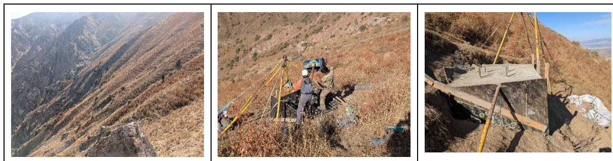
Figure 7: Illustration of the civil works of the O'Belx foundations in the northern slopes (a) undergone with local means in challenging environment (b & c).
