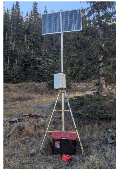
Figure 2: BADS PoE Field Deployment with Base Station
