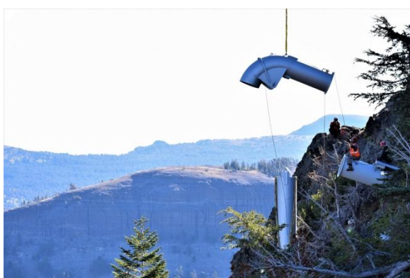
Figure 9: Gazex exploder replacement at Carson Spur, 2022.
