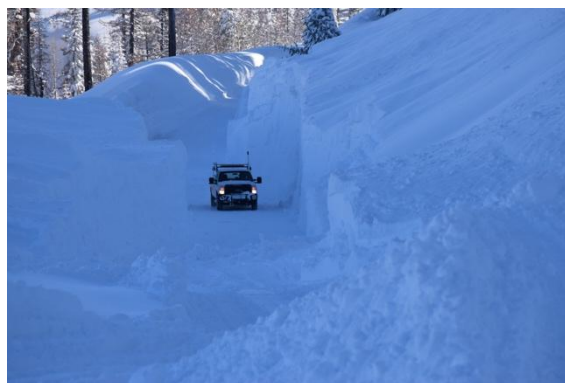
Figure 7: Snow-removal operations at Carson Spur, 2023.
