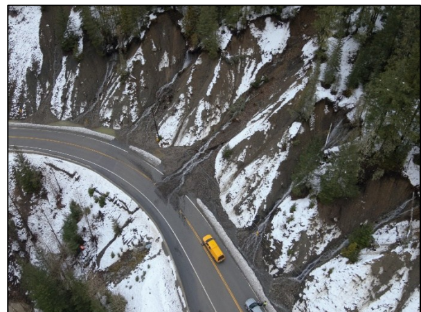
Figures 9 & 10 - New major culvert site 42km (top) and debris flow onto BC Highway 3 (bottom), both on December 19, 2025. Source: BC MoTT Flickr account.
