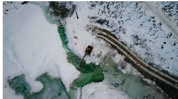
Figure 3: A snow avalanche went into the river Driva in 2018 and formed a plug of snow/ice that dammed the water in the river by 5–6 m. As an emergency measure, a temporary road was made down to the snow/ice plug, so that a trench could be dug in the plug to get a controlled emptying of the dammed river. (Photo: Simon Joachim Oldani, NVE)
