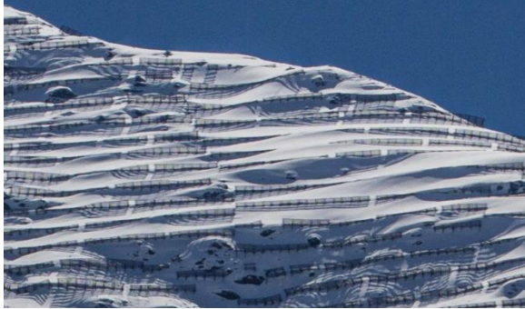
Figure 2: Distribution of snow in release areas when support structures are in place. (Photo: Arni Jonsson)
