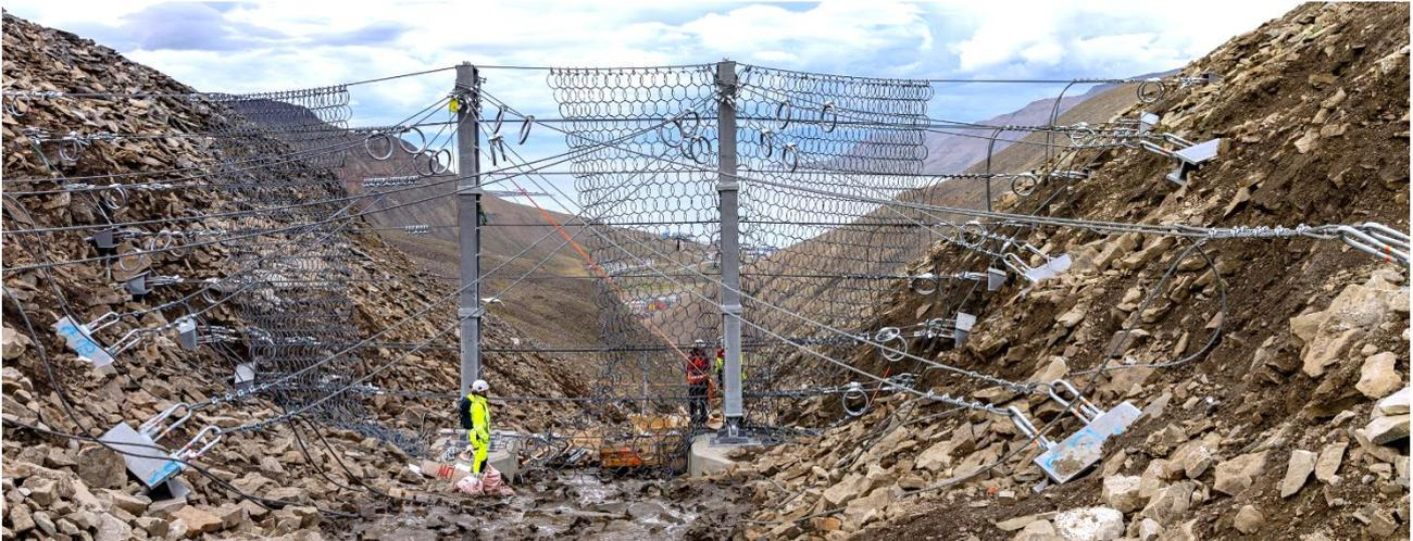
Figure 7 shows installation of 7 m high posts at net 13 on 19<sup>th</sup> of August 2024. The horizontal ropes and retaining ropes are connected to the Flexheads/anchors but the work on the ring net is still under way. The photo also shows how fractured and loose the Svalbard rock and soil is. Photo: Arni Jonsson.
