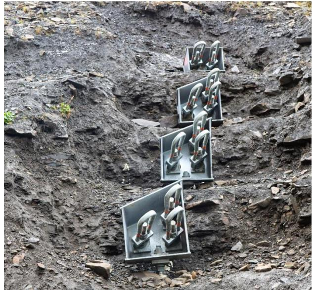
Figure 2 shows 2 and 3-anchor houses used for horizontal anchoring/ropes on side slopes. Photo: Arni Jonsson.
