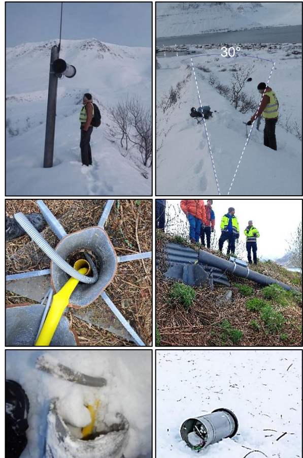
Figure 10: The radar mast. Top: The mast on the lower (left) and upper (right) half of the dam. Middle: The broken mast. Bottom: A close-up of the broken mast on top of the dam and the radar antenna, 280 m downstream from the mast. Photos: K. M. Hákonardóttir, R. Lárusson and G. H. Halldórsson.
