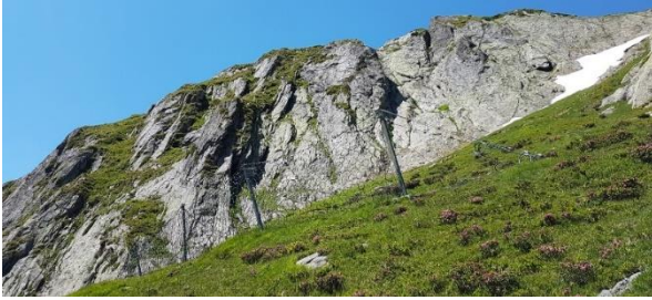
Fig. 6: Rockfall barrier at Rosalba on September 8, 2023.
