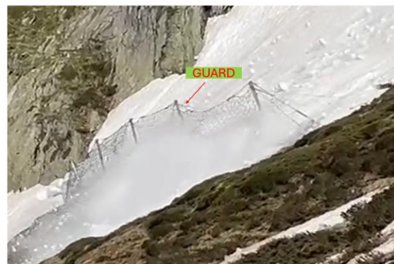
Fig. 15: Documented avalanche impact on the rockfall barrier on June 11, 2024, in Rosalba with highlighted GUARD mounted on the upslope anchor rope.
