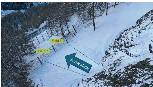
Fig. 9: Rockfall barrier at Arolla on March 7, 2024 with recorded snow slide in field 6 and 7.
