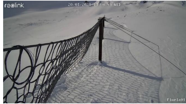
Fig. 3: Snow filled rockfall barrier at Chant Sura in January 2021.
