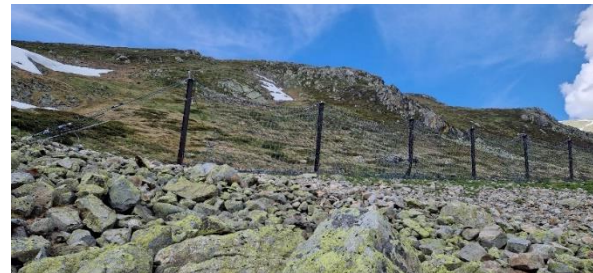
Fig. 4: Rockfall barrier at Chant Sura on June 13, 2023.
