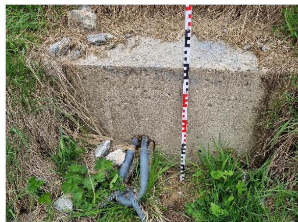
Fig. 19: Proposed uphill concrete anchorage solution for Rosalba.
