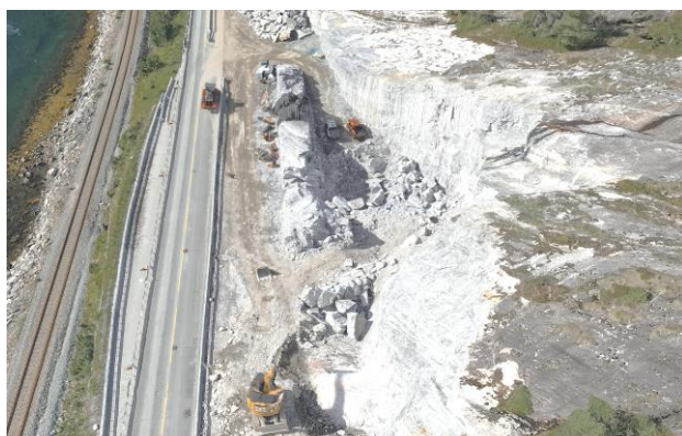
Figure 2: Construction of catchment dams in progress by drilling and blasting. Screenshot from a photogrammetry 3D model.
