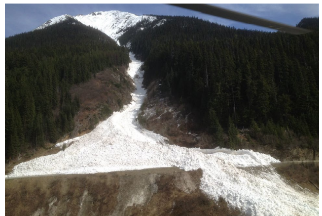
Figure 2: Photo of an explosive-triggered avalanche in Path 51 on May 14, 2012. The highway crosses the bottom of the photo, where most of the debris has accumulated (Source: MoTI).
