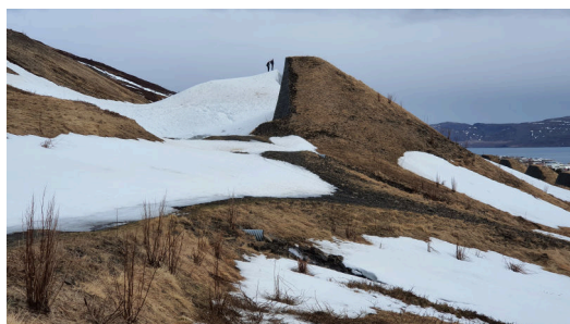
Figure 7: Snow deposit by a braking mound below the Innra-Tröllagil avalanche path in Neskaupstaður from an avalanche on 30 March 2023. Photo: Sveinn Brynjólfsson, 12 April 2023.
