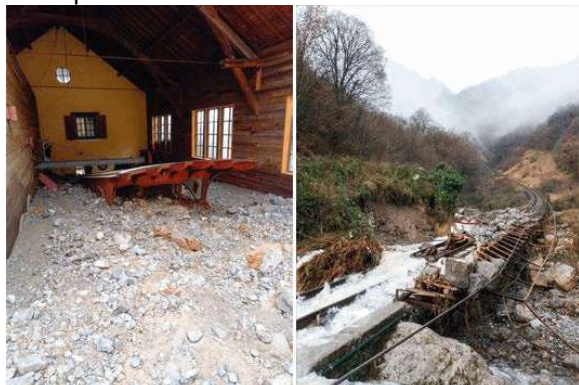
Figure 6 : Impacts of the 29 December 2021 natural disaster (debris flow) around the lower station of the funicular. Right : detached railway. Left : One of the cabin buried under metres of debris. © Radio France - Dominique Clouzeau.
