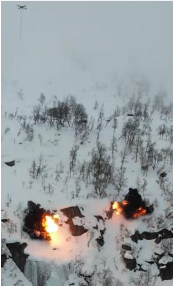
Figure 2: Deployment of multiple charges in the terrain with simultaneously detonations. Photo: AF Decom
