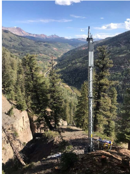
Figure 12: Yellow Springs Gully tower after construction was complete
