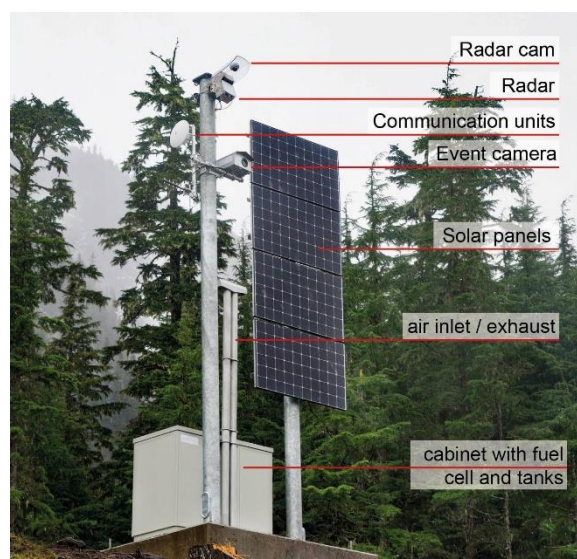
Figure 2: Station design of the autonomous avalanche radar station at Bear Pass, George Copper site.
