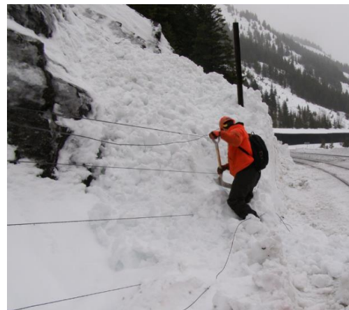
Photo 2: Clearing avalanche debris on a slide fence.
