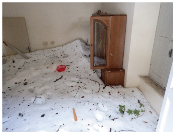
Fig. 10: a room of a house in Foce di Montemonaco (AP). The windows and doors of the 1 st and 2 nd floor on the exposed side were smashed and snow and debris were powerfully injected inside all rooms. Fortunately, the village had already been evacuated [source CFM PC Regione Marche and AINEVA - photo Chiambretti].
