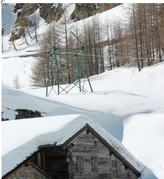
Figure 5. Exceptional avalanche that reached the regional road before the village of Pont in the upper Valsavarenche on January 8 th . Great damages to high voltage power line and to the woods
