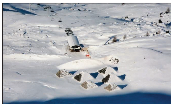
Figure 4: View of the "pyramids" and dam network at the end of 2017
