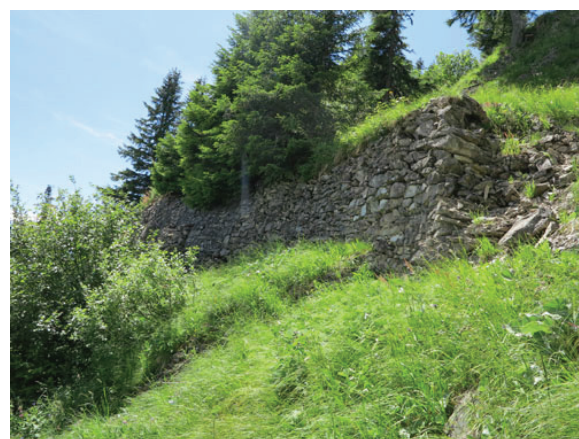
Figure 5: Protection wall with gabion – most important building in the area (IBLB BOKU Vienna, 2018).
