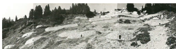
Figure 1: Slope with historical avalanche protection barriers, Kleinwalsertal (WLVV, 1956).
