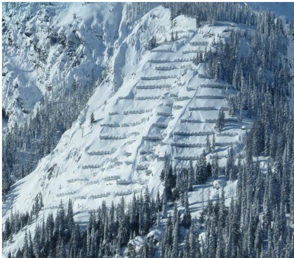
Figure 9: Cougar Corner 7 and 8 path snow nets, March 2018.
