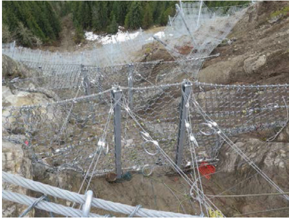
Figure 8: Use of debris flow net barrier in CC7 gully.
