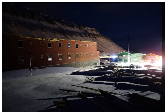
Figure 10: Roof blown off of house in Nybyen. Photo: Kjetil Brattlien, NGI.
