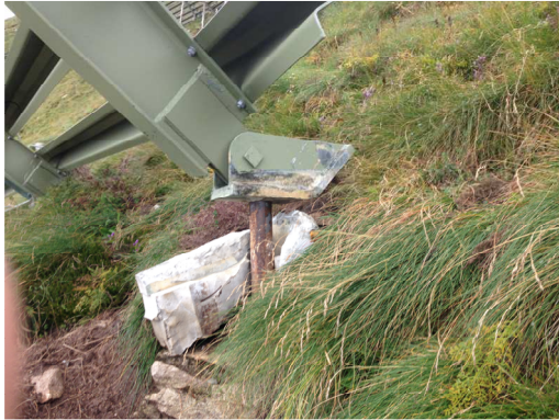
Fig. 6: example of the failure of the foundation plinth on the support of a snow bridge
