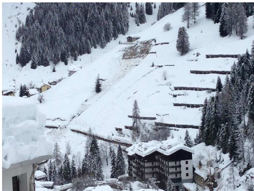
Fig. 2: example of ground avalanche between the lines
