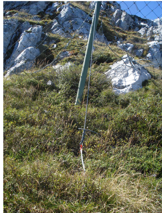
Fig. 5: example of a complete pulling out of a downhill anchor in a snow net
