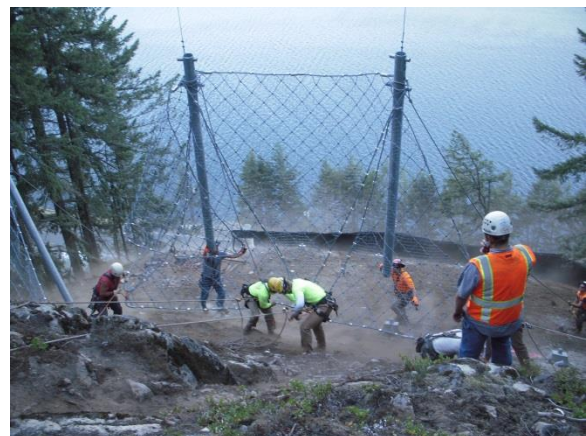
Figure 8 & 9. Helicopter installing post & nets
