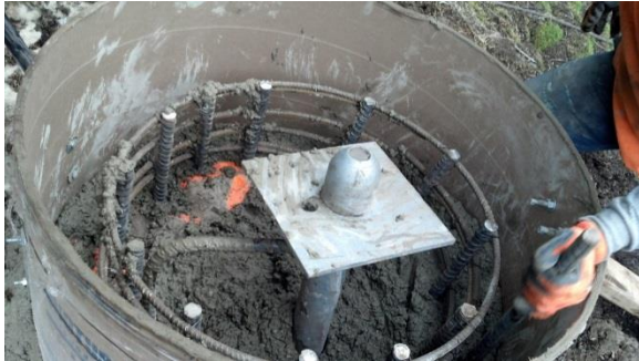
Figure 5. Pier footing being prepared
