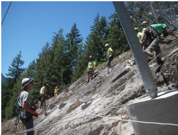
Figure 6. Completed pier footing
