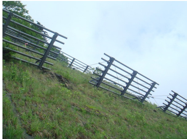
Fig. 7: Snow bridges installed on a slope along a highway in Nakayama pass.
