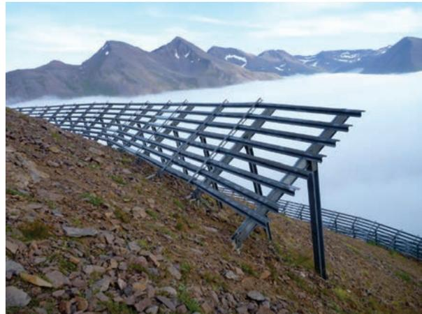
Fig. 7: Steel bridges in the release area Gróuskarðshnjúkur built in 2004. The structure height is 3.5 m and the length of the cross-beams is 4 m (Photo: S. Margreth).
