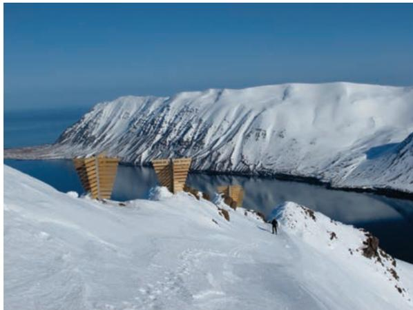
Fig. 8: Wind baffles on the top of Hafnarhryrna on 28 March 2014. The beginning of the large cornice is on the right side of the wind baffles. The wind baffles have not led to a substantial change in the snow distribution in winter 2014 (Photo: T. Jóhannesson).
