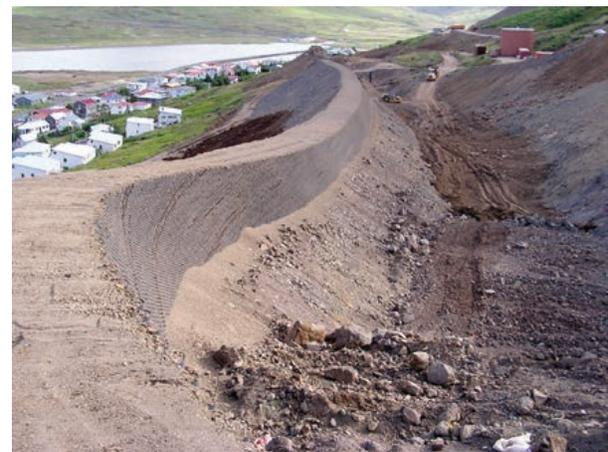
Fig. 6: Catching dam in construction, the steep top section is made of geocells (Photo: Þ. Jóhannesson).
