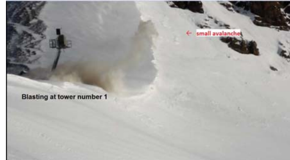
Figure 4. Avalanche measured on April 9th 2012, the location of the avalanche is indicated by the red arrow.
