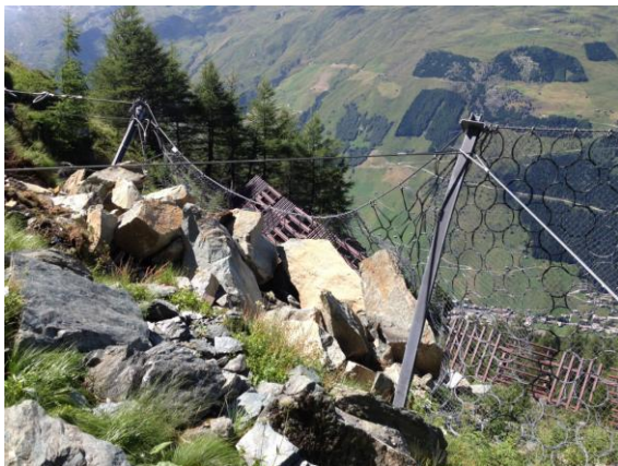
Figure 6. Rockfall barrier above an avalanche defense structure. Most of the blocks were stopped by the rockfall barrier.
