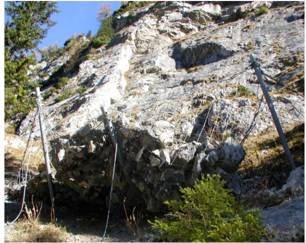
Figure 4. Above the uppermost lines of snow nets is a cliff with a height of more than 50 m from which rockfall can occur. The snow net is heavily filled with caught blocks (Location: Hahnenspiel FL).
