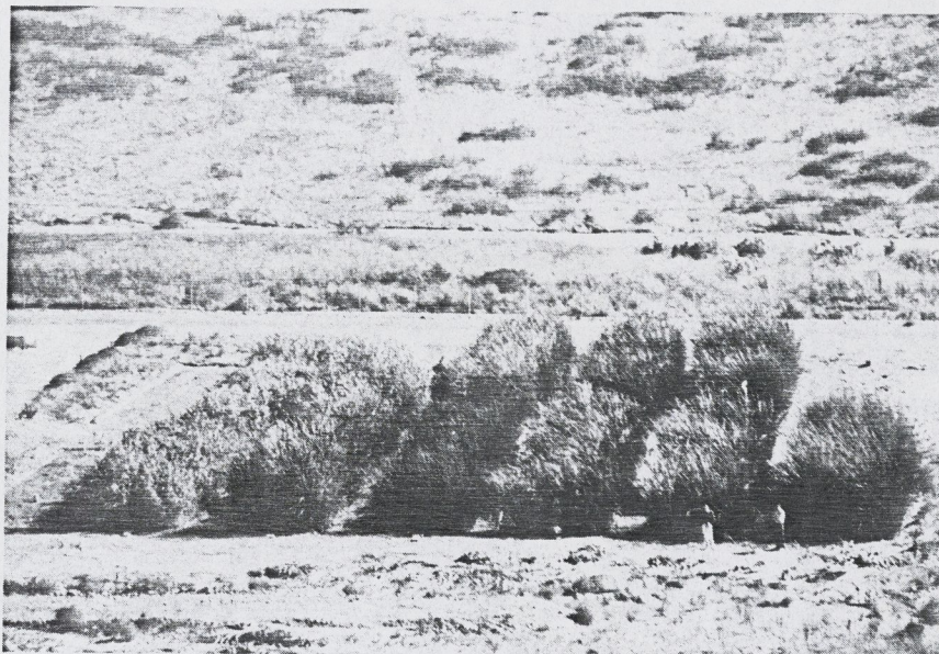
Fig. 1. Photograph of artificial wetlands site at the Santee Water Reclamation Facility. For scale, note the two persons standing at right in foreground. Each of the fourteen marsh beds are 18.5 m long \times 3.5 m wide; vegetation ranges from 3 to 4 m in height. The two unplanted control beds can be seen at the extreme left.
