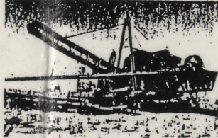
Dry land dredge operated on east bank below Green River in 1890s, recovered little gold.
