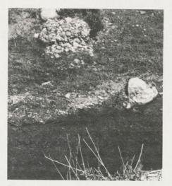
Figure 9. Eroded gabion, Big Creek.
