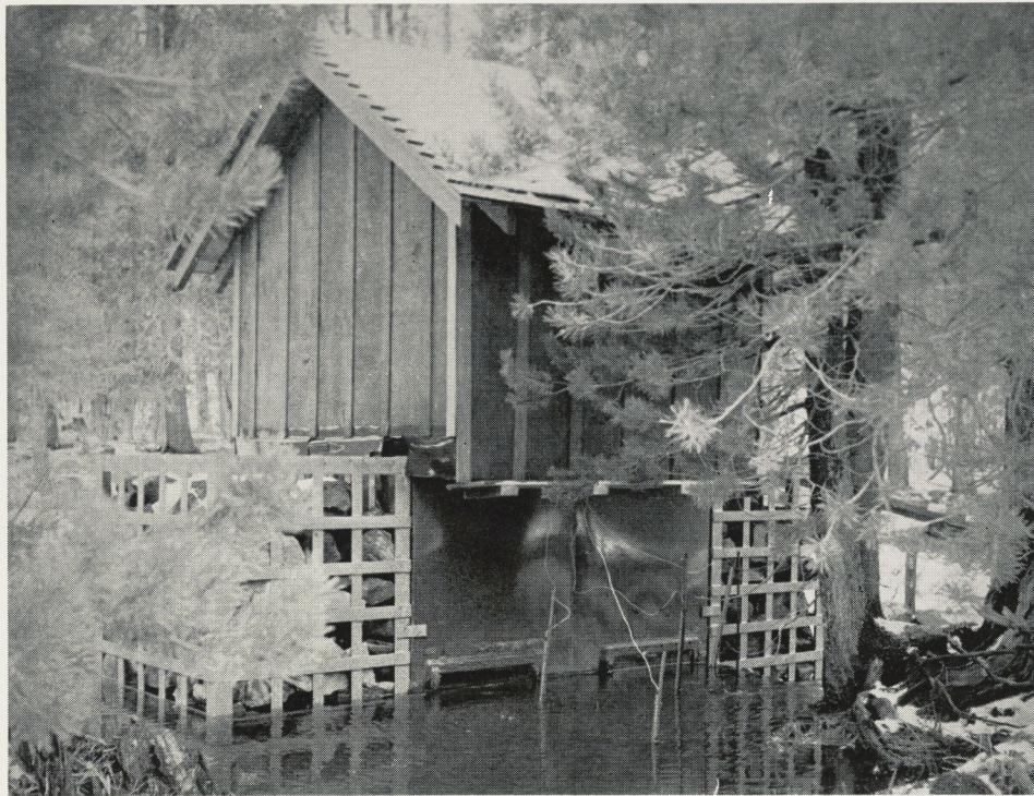
FIG. 2. Underwater observation tank at the Sagehen Creek Project. Rock racks at each end counteract buoyancy. The tops of two of the viewing windows show just above the water surface. The rods in the pool hold thermocouple stations in position for temperature studies. Access is by ramp at right of photo.
