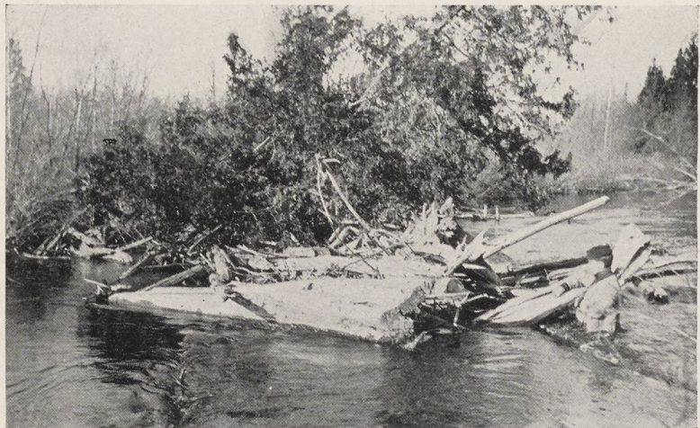
A splendid trout hole has been added to the stream by the installation of a deflector on the Pigeon River. Note the apparent depth of the hole dug by the artificially deflected current.
