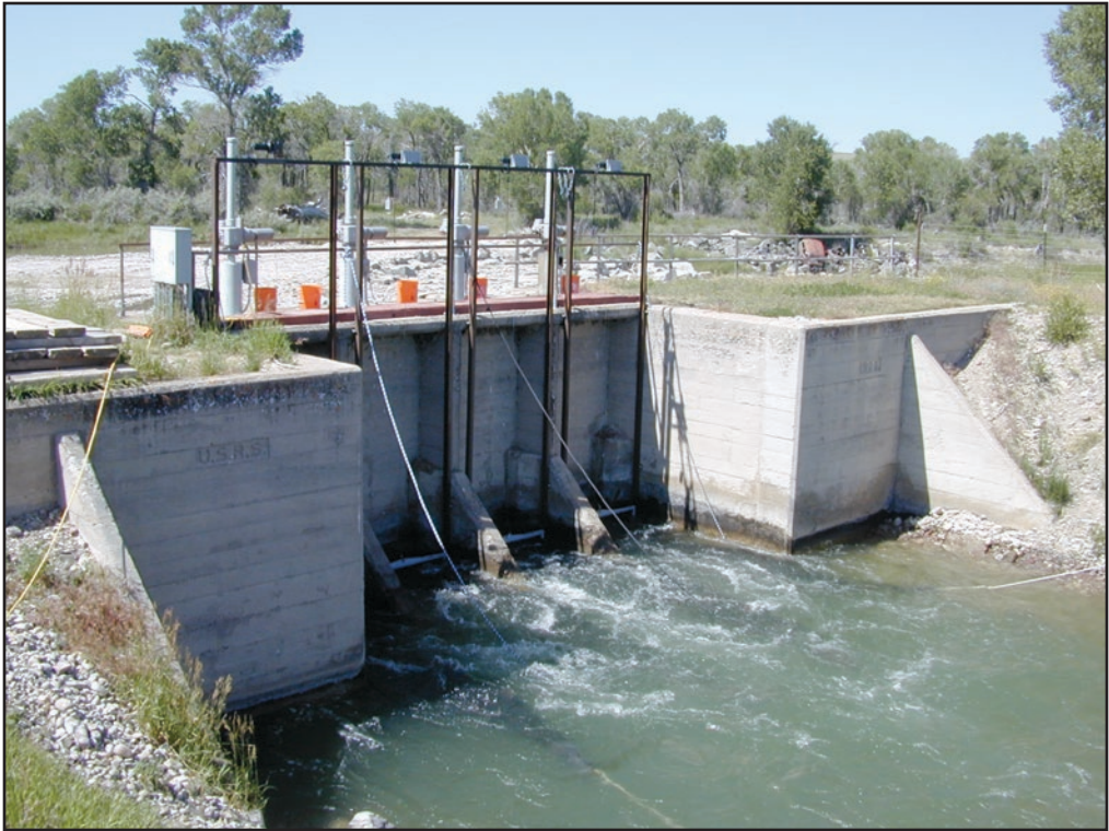
Figure 3. Photograph of the deployed Fort Shaw Diversion entrainment netting system. Aspect is from the canal side.
