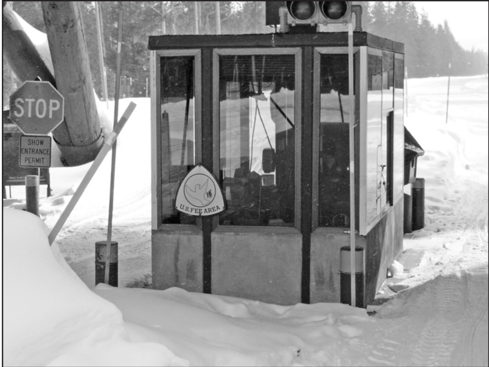
Figure 1. Kiosk used by employees to supervise snow machine traffic entering YNP through its West Entrance.
