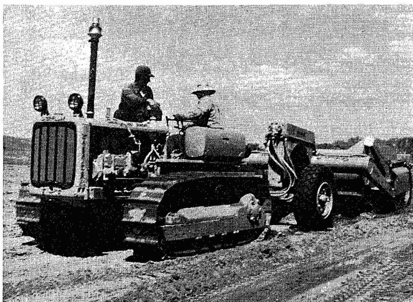
Figure 16—Heavy dirt moving equipment is available through contractors and soil conservation districts
