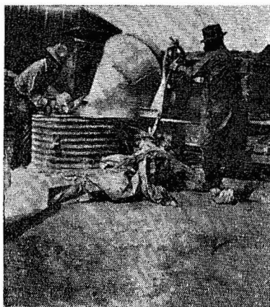
Figure 3. Emptying mixed dust from mixer. Notice platform for refilling in background.
