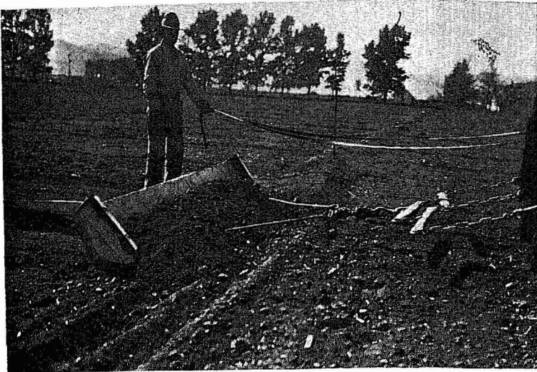
Fig. 17—Homemade buck scraper or fresno for building border dikes.
