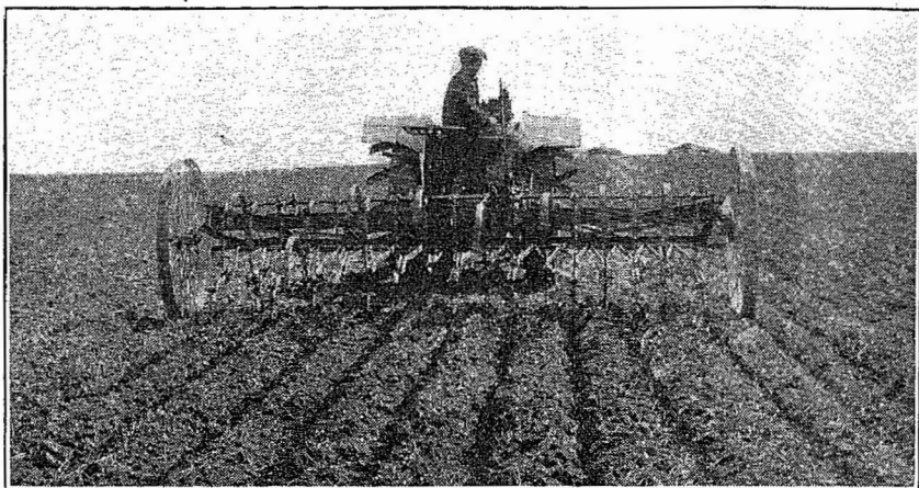
Fig. 9—A duckfoot cultivator in action on "plowless" summer fallow. Note the clods and rubbish on the surface: Attention is called to the homemade spring teeth, sometimes used to level the ridges.
