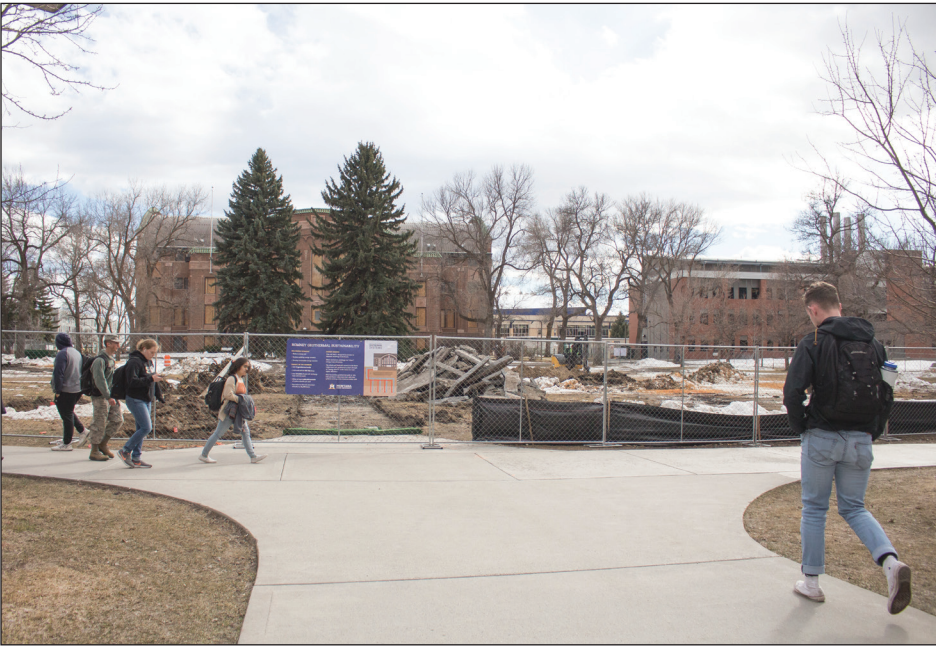
Students pass by the debris from pavement and tree removal in Romney Oval as a result of the geothermal energy project being undertaken by MSU. PHOTO BY MARIE STEIGER
